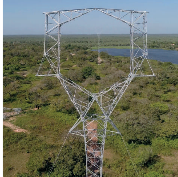
Electricity tower of the Brazilian company Argo, which is in the process of being acquired
