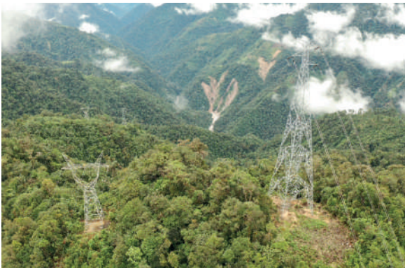
After a lot of hard work, the tower was raised, which enables the transportation of electric energy to southern Colombia
