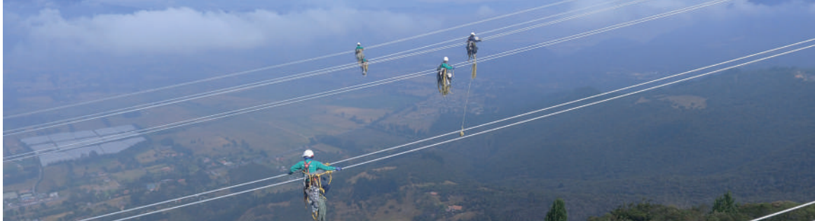
Transmission line maintenance at Guavio-Circo
