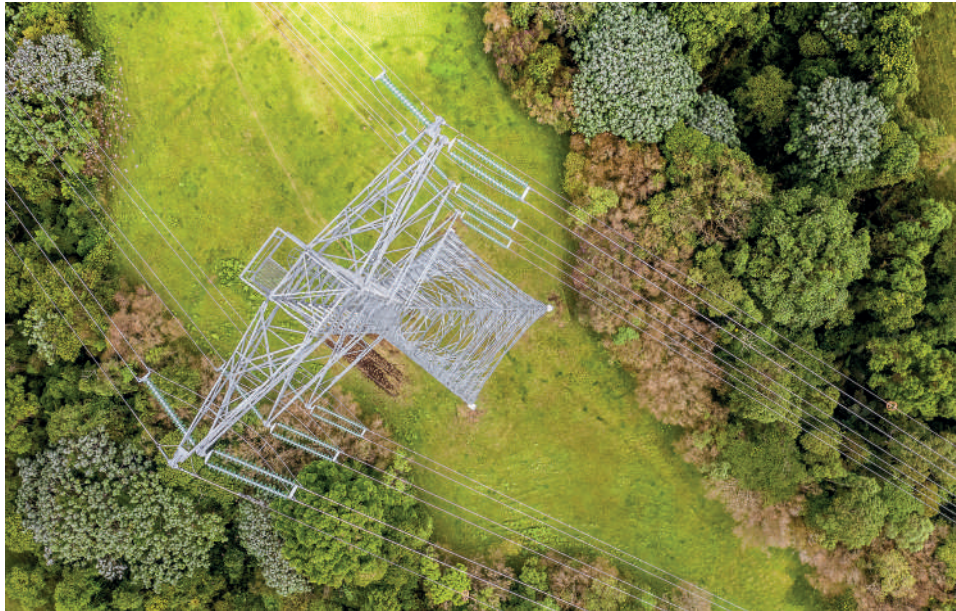
Transmission tower in the Filandia municipality, part of the Armenia project between the Quindío and Risaralda departments.
