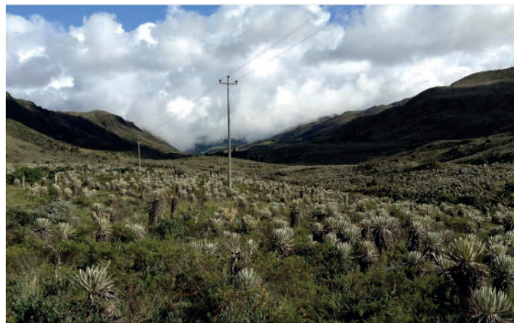
Transmission tower in Filandia municipality, part of the Armenia project in the departments of Quindío and Risaralda.
